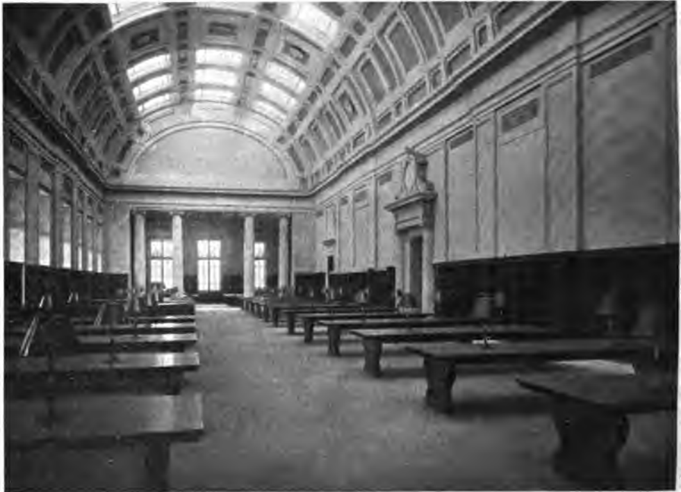
GENERAL READING ROOM, OCCUPYING FRONT OF SECOND FLOOR.
